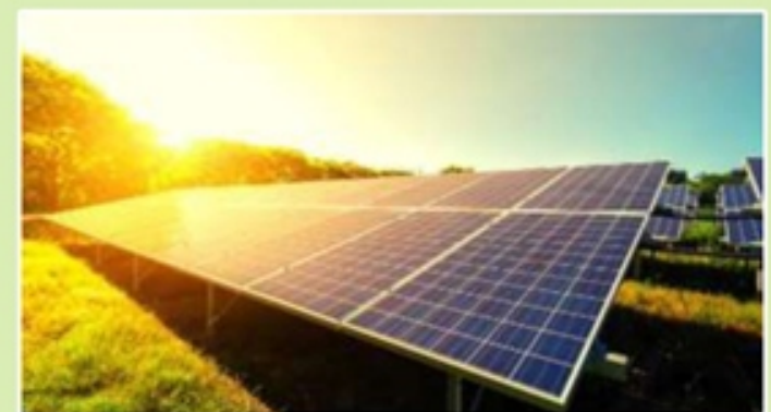
WORLD 'S LARGEST SOLAR PARK OF 5,000 MW
