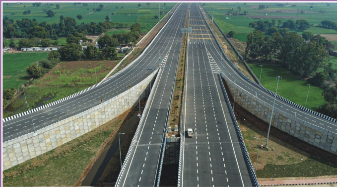
New Six lane Express Way
