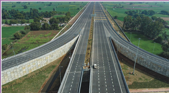
New Six lane Express Way
