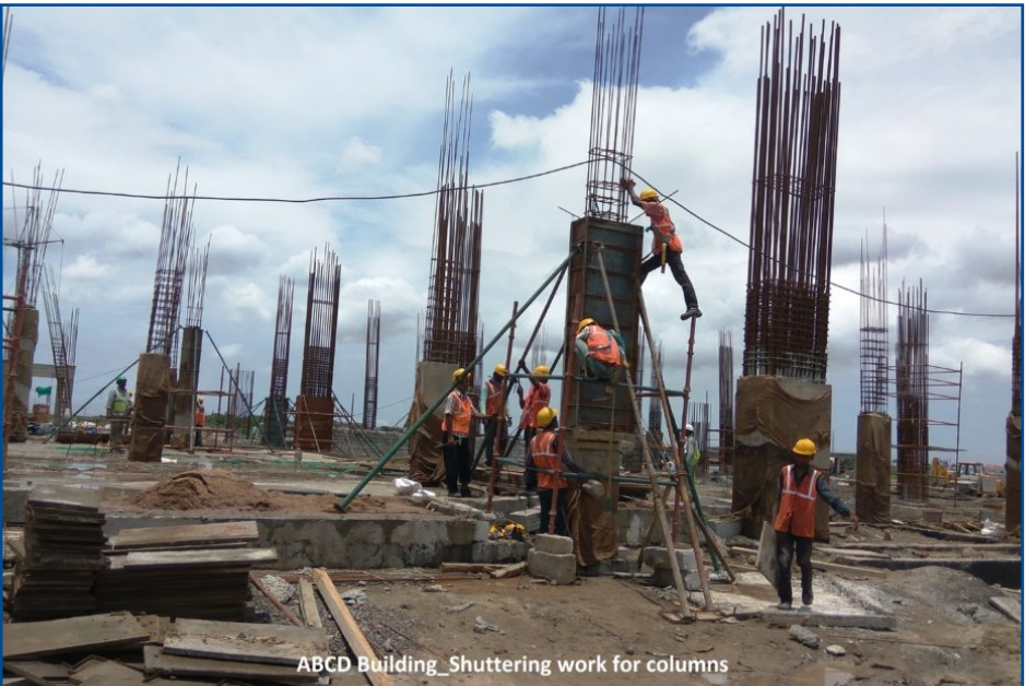
ABCD Building_Formwork
