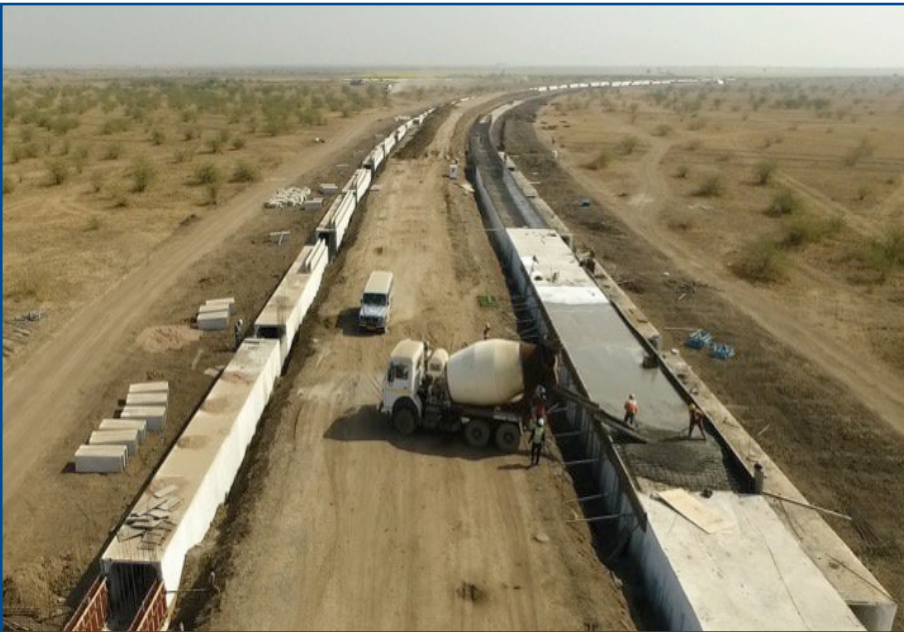
Bridge Foundation Concreting for Raft
