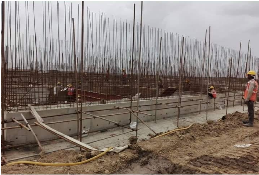
STP_Anoxic & Aeration tank wall 1st lift
