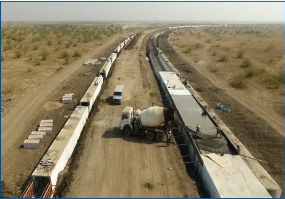
Bridge Foundation Concreting for Raft
