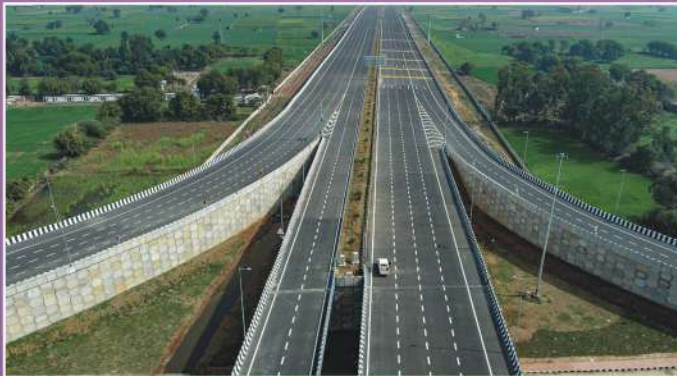
New Six lane Express Way
