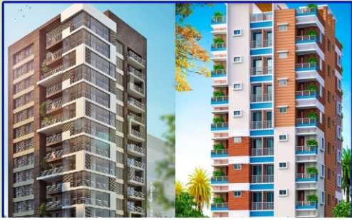
Residential multi storey apartment
