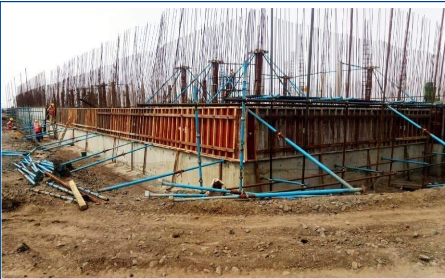
STP- Anoxic & Aeration tank shuttering work in progress
